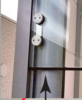
D-pad installed on door edge
