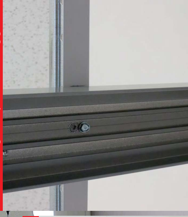
Attaching track piece to ceiling grid
