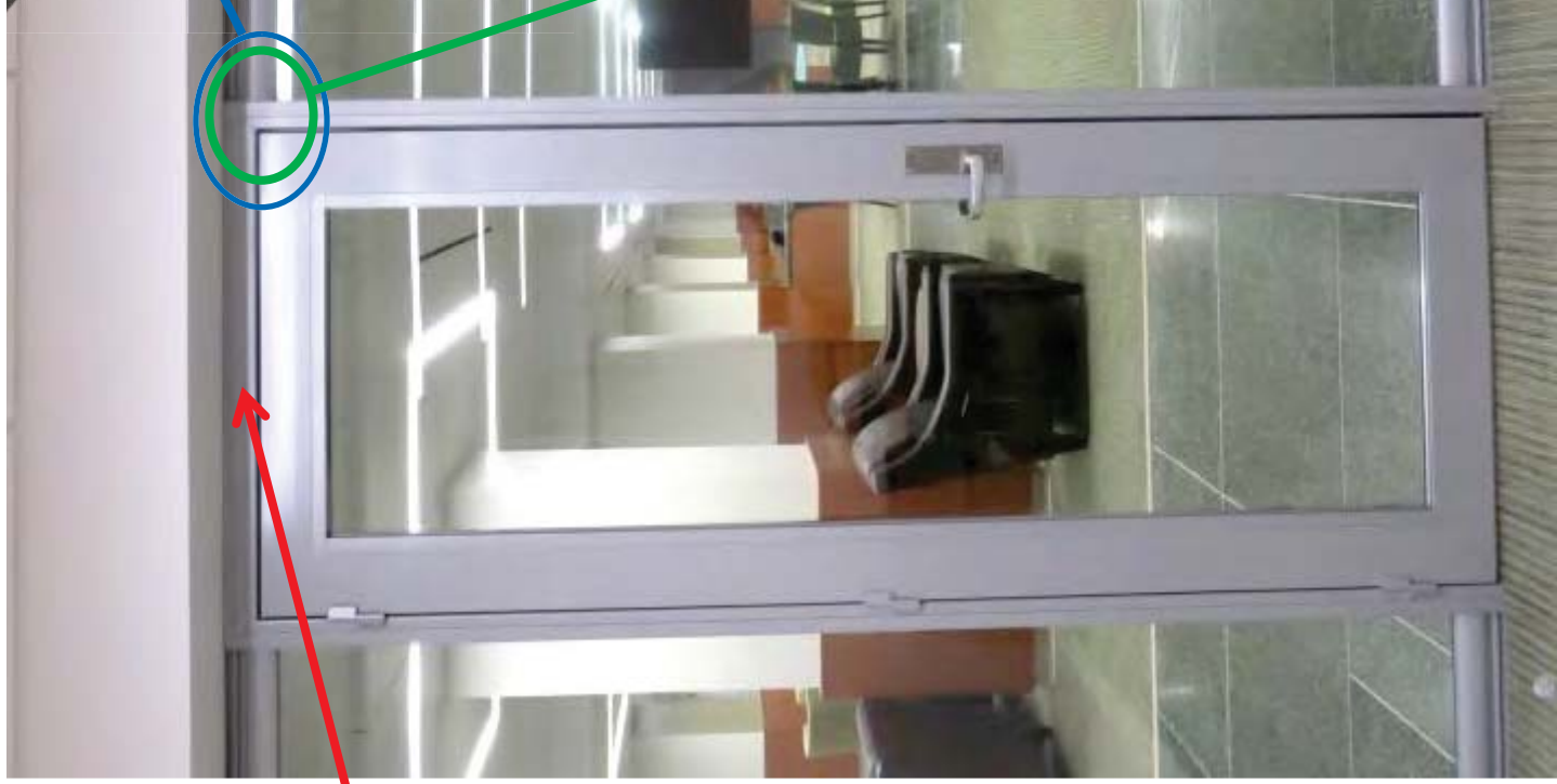
Detail Image: T-bracket installed with a Wall Start, Flex Track, and View Track.
