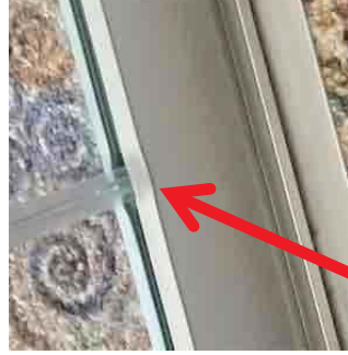
Spline Notch-out Detail
