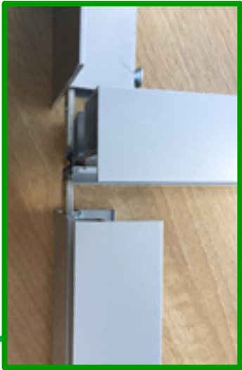
Detail Image: T-bracket installed with a Wall Start, Flex Track, and View Track.
