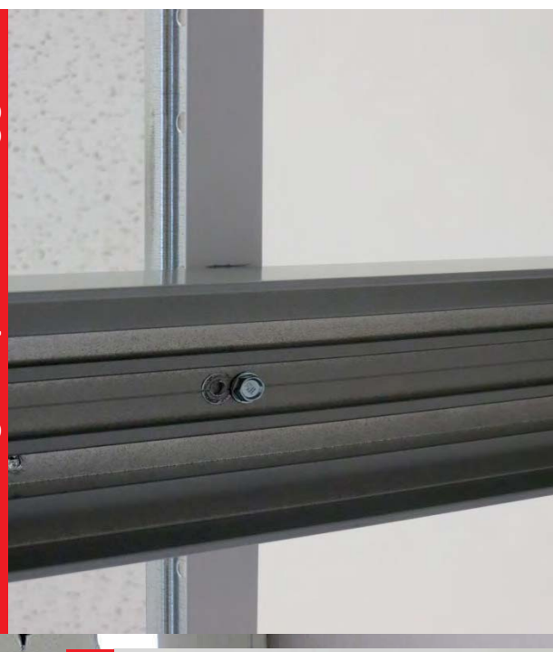
Attaching track piece to ceiling grid
