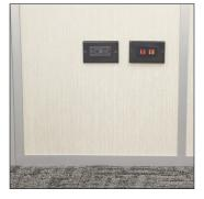
Modular or conventional power and data not confined to raceways.
