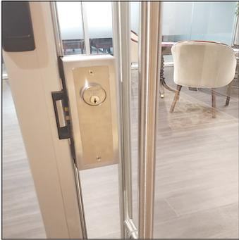
Custom door hardware options such as integrated electronic strike and card reader adds security or traffic control where needed.
