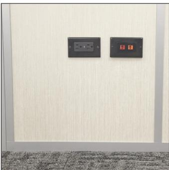
Modular or conventional power and data not confined to raceways.
