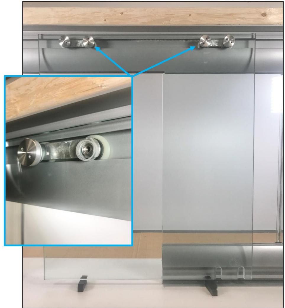
Install the Carriage Caps with Washers onto the Carriage Frames going through the door. Tighten the Carriage Caps with a spanner wrench. Avoid overtightening the Carriage Caps, for overtightening will prevent the door from sliding smoothly.
