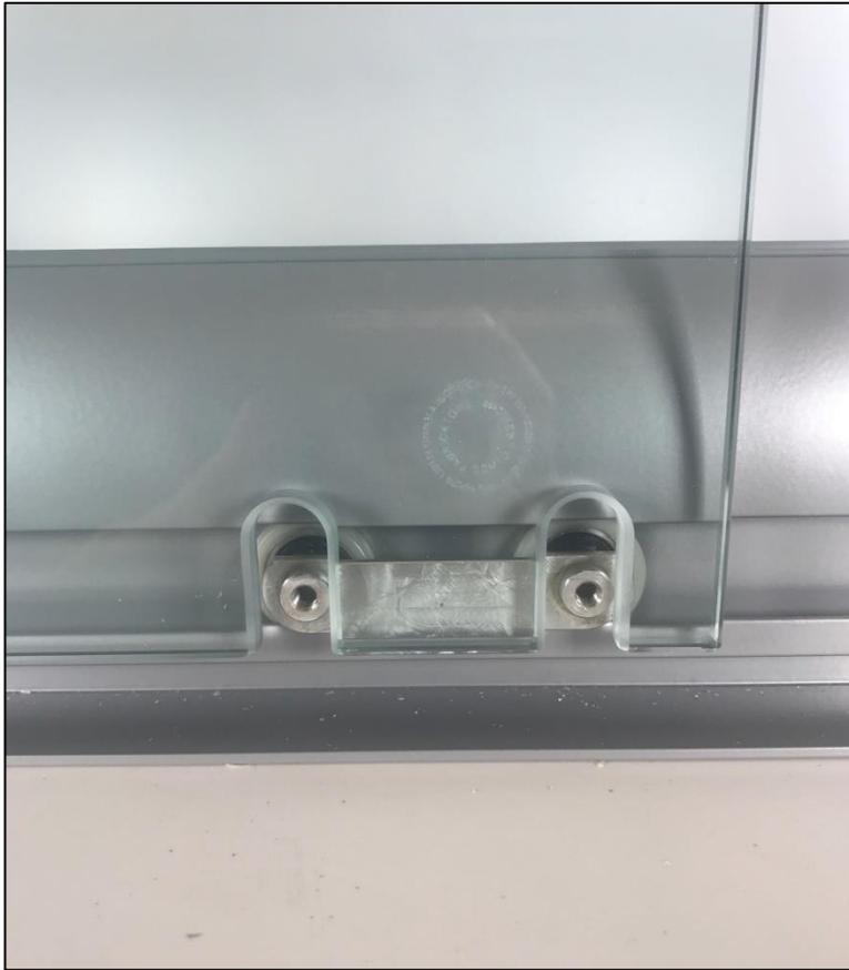
On View Series Frameless Sliding Glass Doors there is a horseshoe shaped cutout at the bottom of the door. A Carriage assembly will be installed in that location. To install the Carriages, repeat the installation process used for the top of the door.
