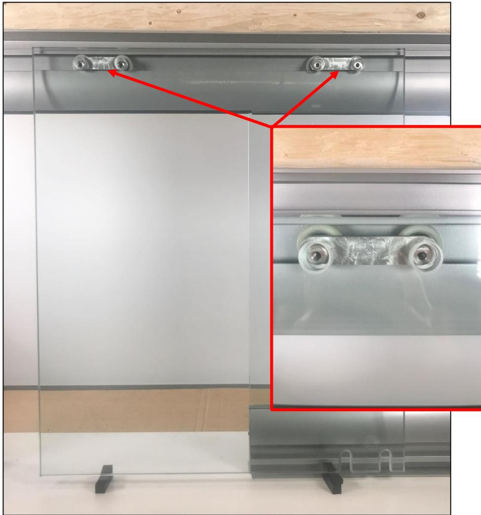
With the Carriages already in the View Track, place the glass door on shims to align the holes in the door with the Carriages. Press the door tight to the View Track to allow the Carriages to go through the holes, as shown above.
