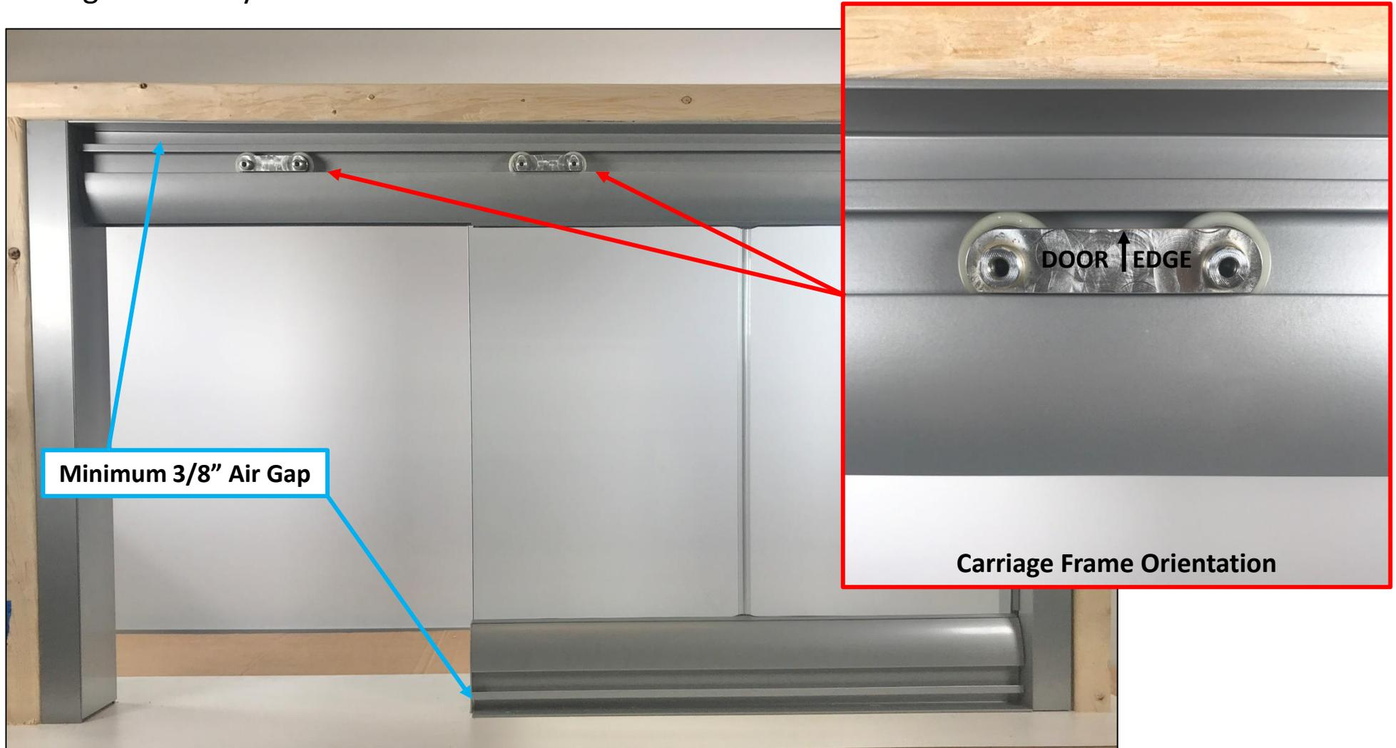
Prior to installing the door make sure the minimum 3/8" air gap is installed between the View Track and Guide at the ceiling and the floor. If the gap is not installed the door will not function properly.
