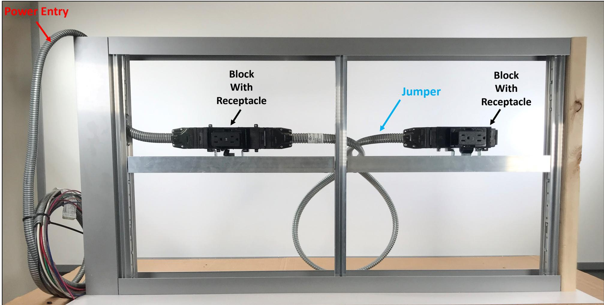
Run the Power Entry and Jumper feeds through the determined locations and connect to the electrical blocks. The Power Entry/Jumpers simply plug into the electrical blocks. Jumpers are used to connect one electrical block to the other.
