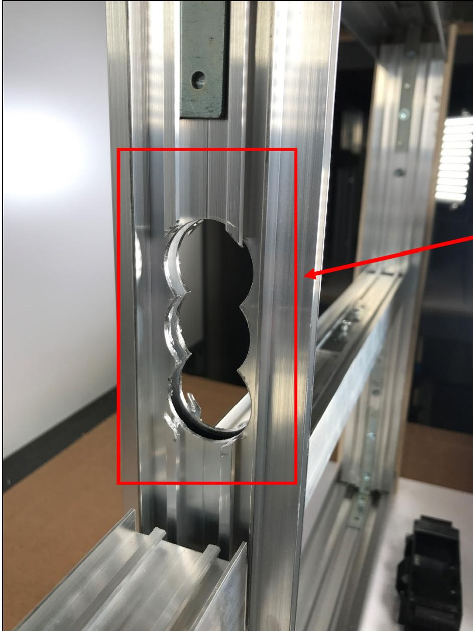
In the locations where the Power Entry and/or Jumpers are needed to pass through a Post/Flex Stud or Flex Stud a hole will need to be drilled out to allow the heads of the Power Entry and/or Jumpers to be brought through.
