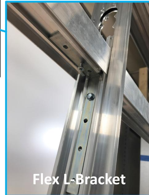
Reinforced studs are only needed at the electrical locations. Cut the Reinforced Studs to fit between the vertical Flex Studs. Cut the Reinforced Studs a 1/4" short, leaving a small gap to avoid bowing the vertical Flex Stud. Slide two Flex L-Brackets into the bottom side of the Reinforced Stud. Prior to attaching the L-Brackets, slide the Track Joiner in the top side of the Reinforced Stud.
