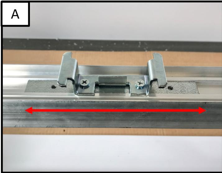
**A:** Attach the Raceway Bracket to the Track Joiner. Use the set screws already installed in the Track Joiner. The Track Joiner & Bracket can be slid side-to-side until it is in the desired location. Tighten the set screws to fix in place.
